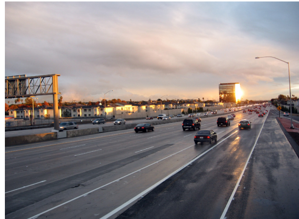
Major highway projects in California include Route 405 in Culver City, CA, where teams expanded and improved five miles of highway and bridges.
